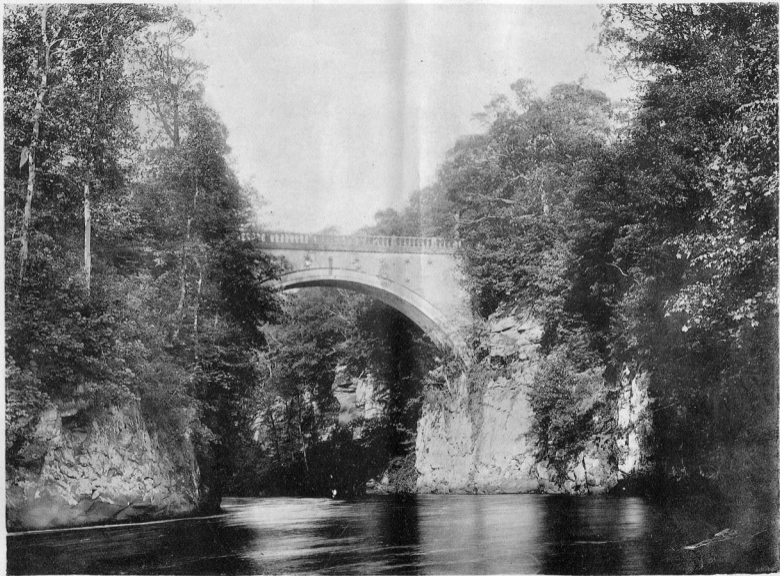
Bridge at Barskimming.—Mauchline.
