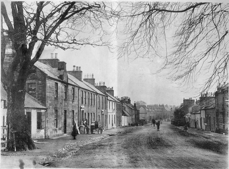
New Road, Mauchline.
